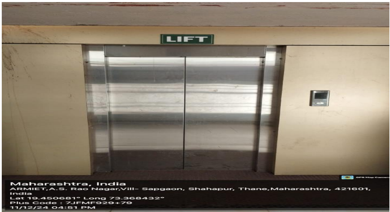
Barrier free access to lift
